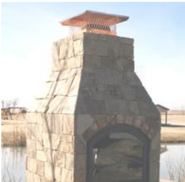
Figure 12. Install Top Cap
