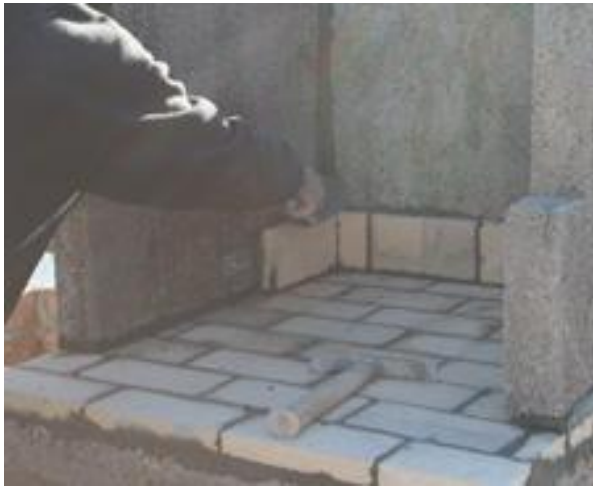
Figure 7. Line Box with Brick
