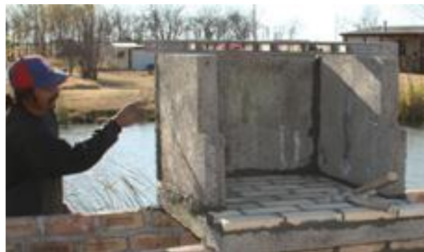
Figure 6. Set Side Walls and Back Plate
