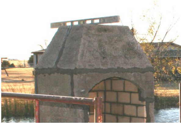
Figure 8. Set Throat and Flue
