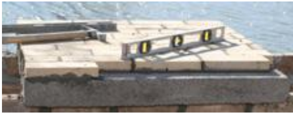
Figure 4. Install Firebrick on Baseplate
