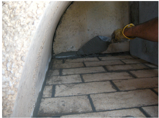
Figure 14. Mortar Inside Joints
