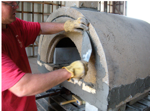
Figure 15. Install Front Wall
