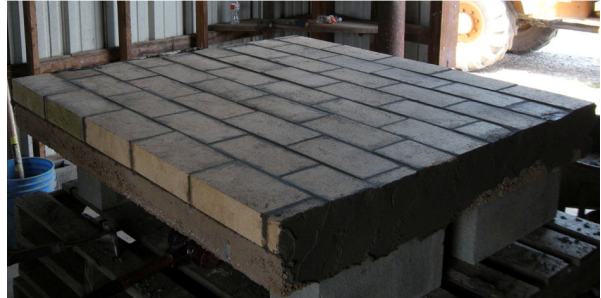
Figure 10. Install Firebrick on Baseplate
