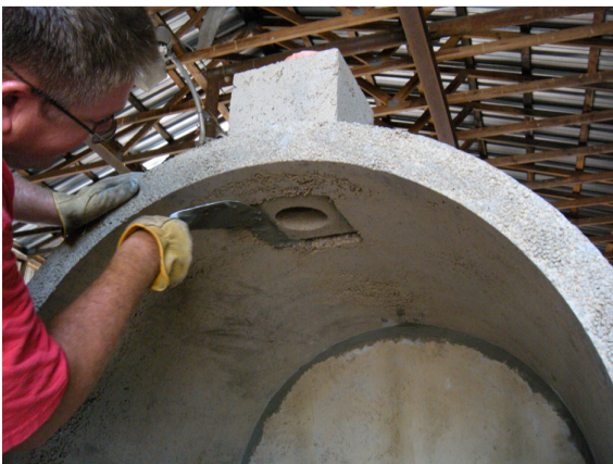
Figure 13. Mortar Chimney Inside of Oven
