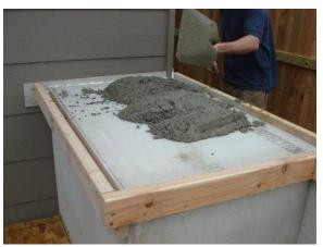
Follow the mixing directions on your concrete mix and then pour the mix into your mold. Be sure to constantly vibrate your mold in order to get rid of trapped air. Tapping it with a hammer will usually give sufficient vibration if you have made the mix to the right consistency. You want to pour the entire top at one time to make sure that you don't end up with any seams.
